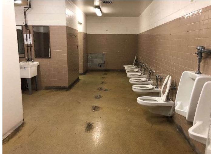
Figure 32: Renovations beginning in old locker room area
